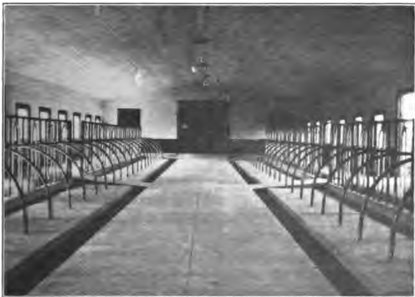
FIGURE 7. —Interior of a good dairy stable. Construction, equipment, lighting, ventilation, etc., of this kind make it easy to keep the floor, walls, ceiling, and stable fittings clean and sanitary
